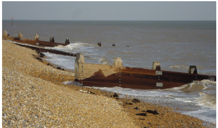
Groynes deflecting the waves on Kingsdown beach © Caroline Millar
