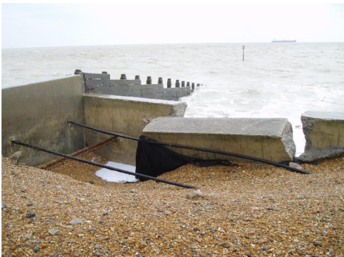
Damage to beach defences at Kingsdown caused by storms and coastal erosion © Helen Williams
