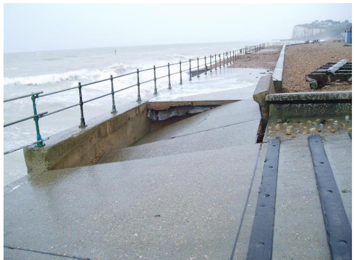
Damage to beach defences at Kingsdown caused by storms and coastal erosion © Helen Williams
